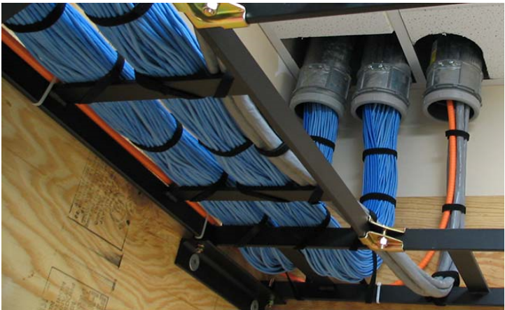
Image: Telecommunications Cabling installed in conduit sleeves and cable tray
